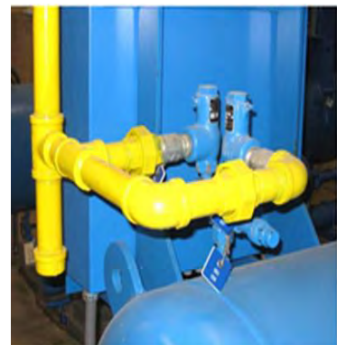
Figure 4: Typical Relief Valve Piping
